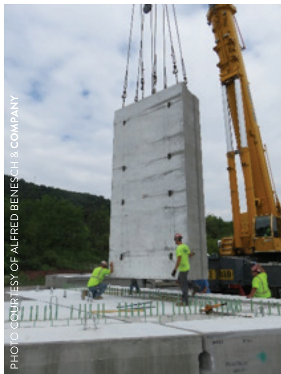
FIGURE 4. PREFABRICATED CONCRETE ABUTMENT
