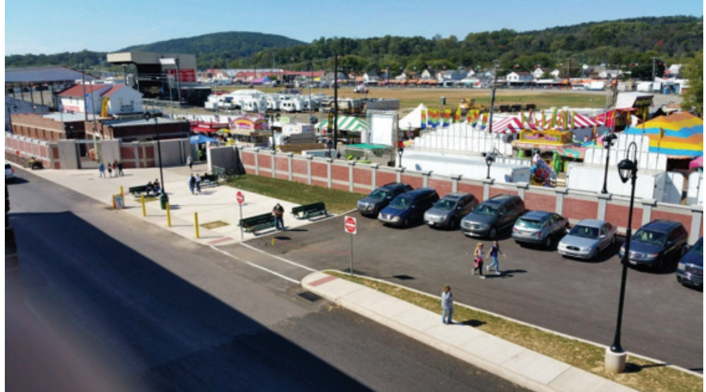
FIGURE 1. BLOOMSBURG LEVEE SYSTEM COMPLETED IN 2015
